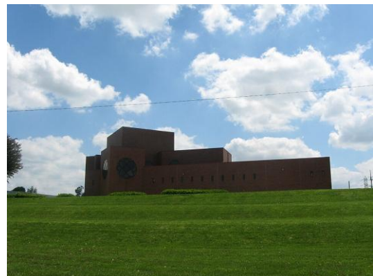
NAIT / ISNA headquarters in Plainfield, Indiana.
